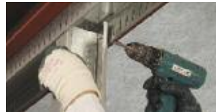
Stud being fixed to slotted head track.
